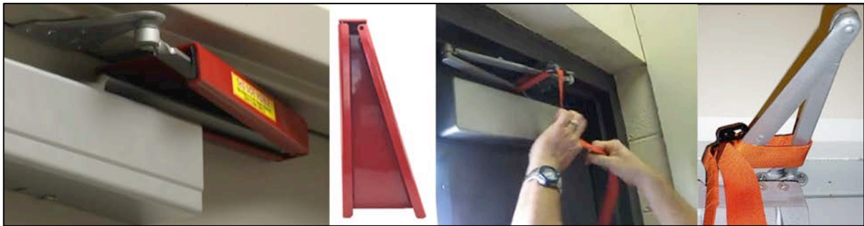
Figure 3-13 Examples of Metal Sleeve and Strap Options to Prevent a Hydraulic Door from Opening
